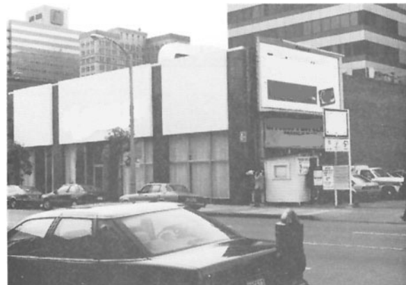
Figure D-8 A 1970s renovated facade hides a URM bearing-wall structure.
