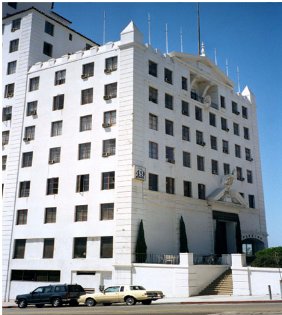
Figure E-21 Concrete shear wall on building exterior.
