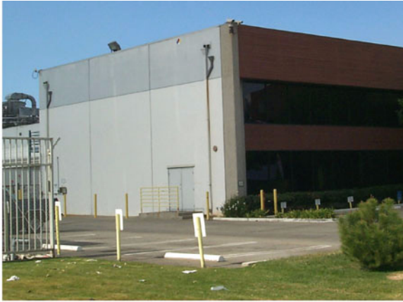
Figure D-5 Regular, full-height joints in a building's wall indicate a concrete tilt-up.
