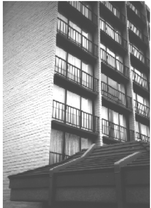
Figure D-7 Reinforced masonry building with exterior wall of concrete masonry units, or concrete blocks.
