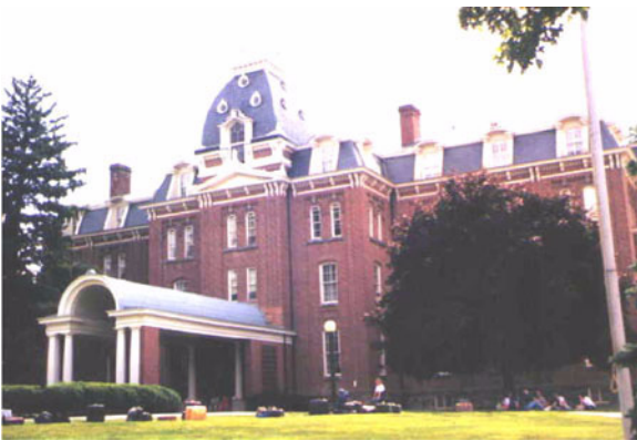
Figure E-50 East coast URM bearing-wall building.
