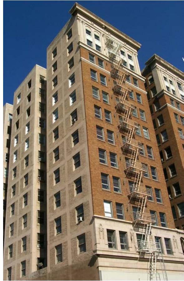
Figure 5-9 Exterior view of 3711 Roxbury.
