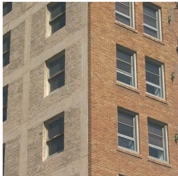
Figure 5-10 Close-up view of 3711 Roxbury Street building exterior showing infill frame construction.
