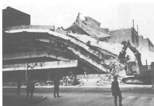
Figure F-5 Mid-rise building collapse, 1985 Mexico City earthquake.
