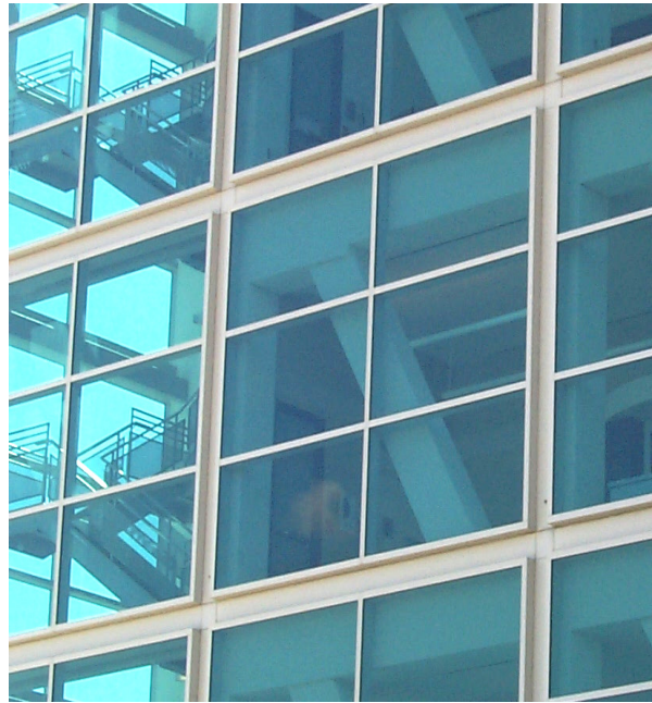
Figure 5-6 Close-up view of 3703 Roxbury Street exterior showing perimeter braced steel framing.
