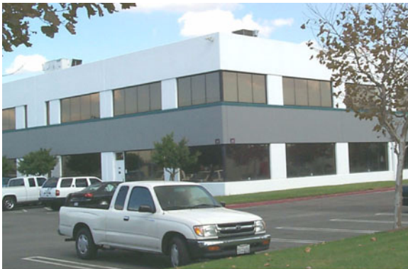
Figure E-37 Tilt-up industrial building, mid- to late 1980s.
