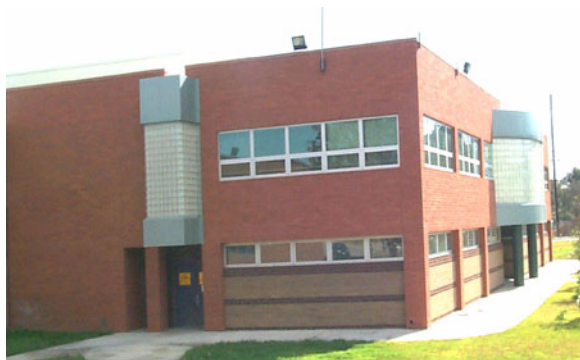
Figure E-46 Modern reinforced brick masonry.
