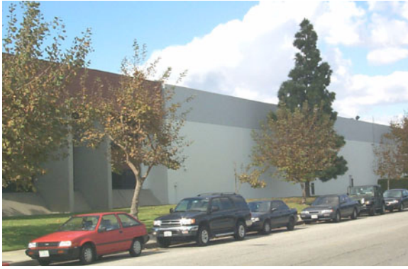
Figure E-36 Tilt-up industrial building, 1970s.
