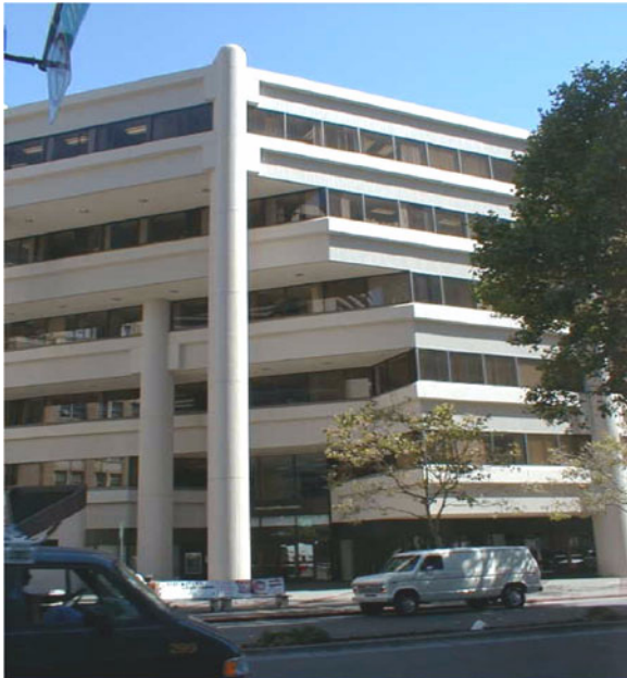
Figure D-2 Building with exterior columns covered with a facade material.
