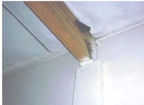
Figure E-40 Newly installed anchorage of roof beam to wall in tilt-up building.
